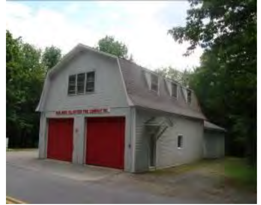
MARLBORO FIRE STATION
