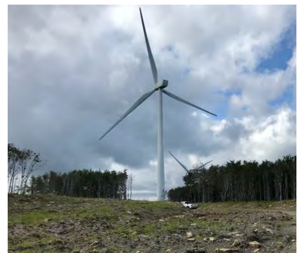
DEERFIELD WIND INSTALLATION, SEARSBURG & READSBORO Photo Credit: WRC
