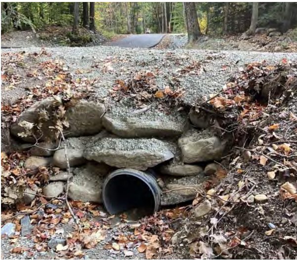
EXAMPLE OF ROAD CULVERT Photo Credit: WRC
