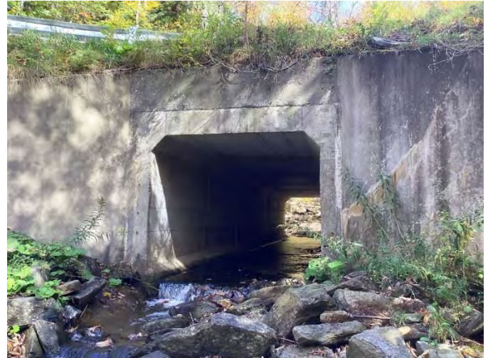
EXAMPLE OF BOX CULVERT Photo Credit: WRC
