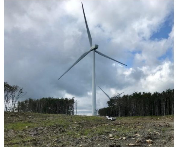
DEERFIELD WIND INSTALLATION, SEARSBURG & READSBORO Photo Credit: WRC
