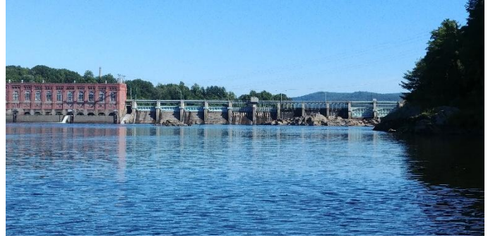
DOWNSTREAM OF VERNON DAM AND HYDROELECTRIC FACILITY
