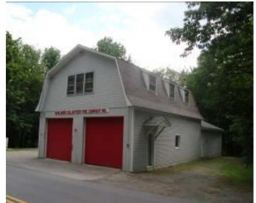
MARLBORO FIRE STATION
