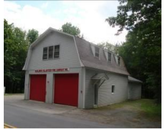
MARLBORO FIRE STATION
