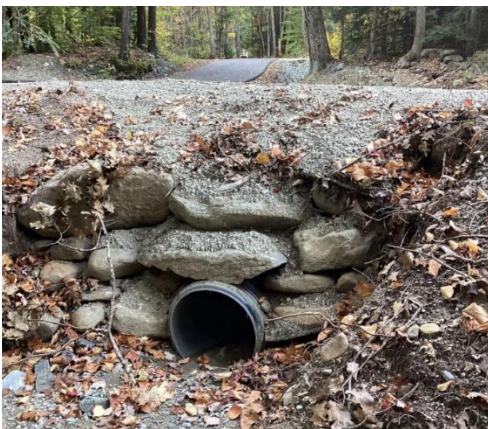
EXAMPLE OF ROAD CULVERT Photo Credit: WRC
