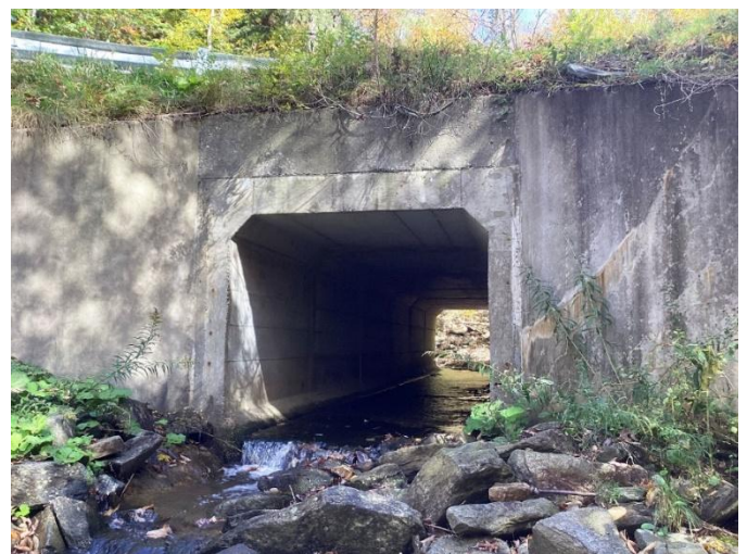
EXAMPLE OF BOX CULVERT Photo Credit: WRC
