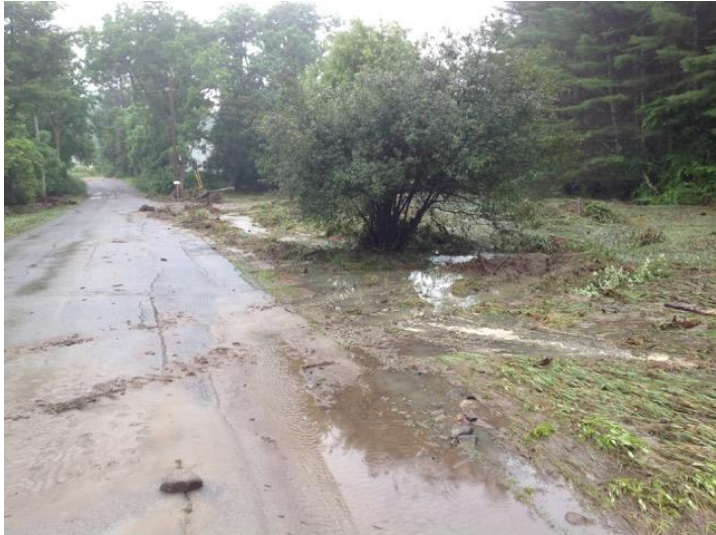
Hill Road damage
